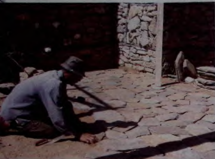
Left: Bricklayer Sakkie Rittmann puts the finishing touches to the outside paving. Behind him are gabions - wire baskets filled with rubble from the Petersen Flats. Far left strip: Old tyres used to make fireproof walls for the Habitat archives. Right: The office block under construction.
